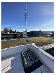
Figure 4-1. Anemometer located on the southern corner of the facility roof.
